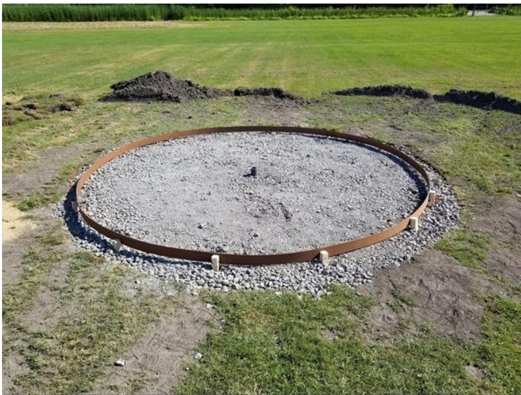
The crew again worked the UCC pour area on Friday and Paul made the 10 foot diameter form:
